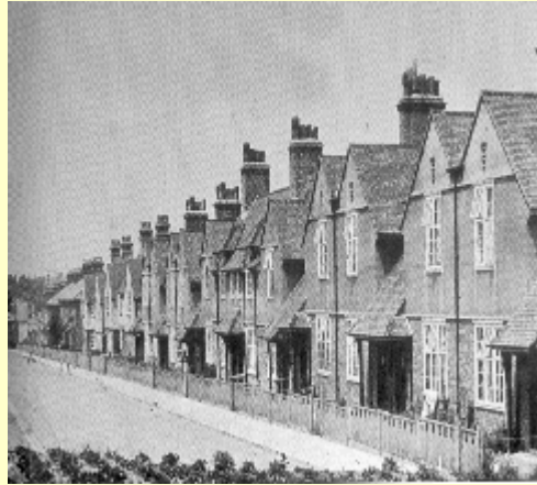
Cline Road was to become the centre of the Jubilee Celebrations of 2002
